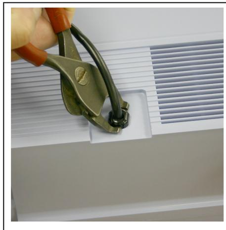
**FIGURE 8-4: STRAIN RELIEF REMOVAL**
